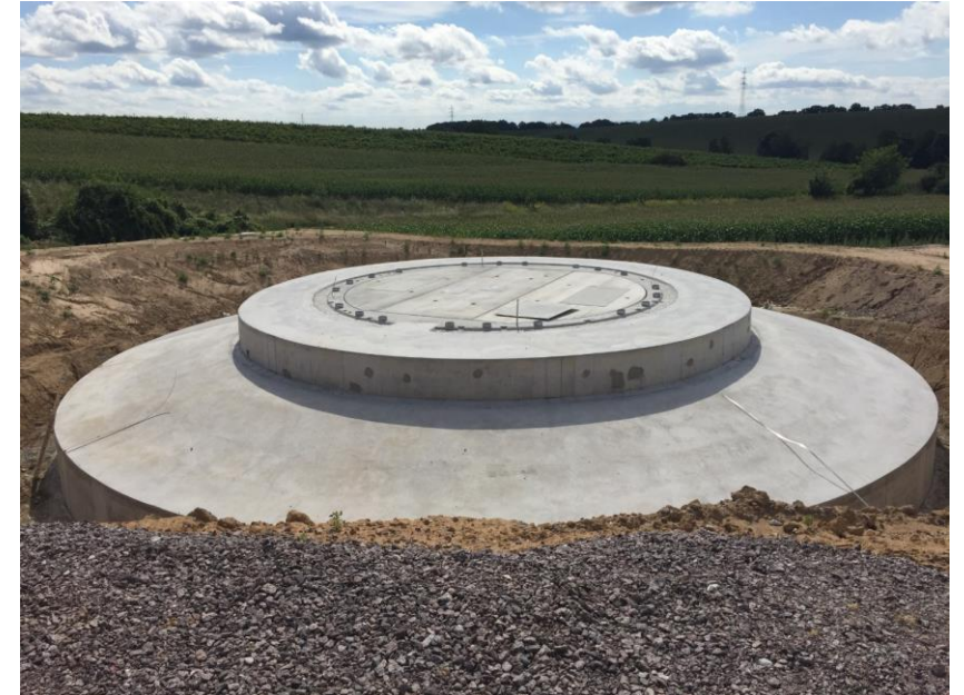
Windpark Hasel - Fundament
